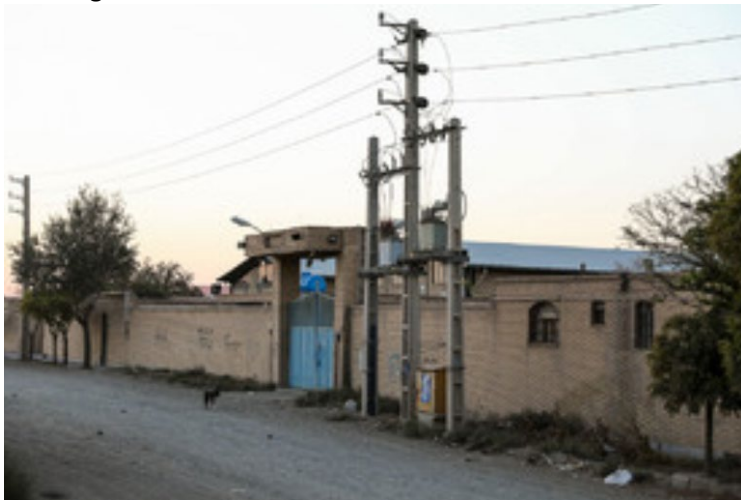
Figure 7. Another image of the front gate of the Atomic Warehouse, showing electrical poles and equipment not visible in front of the carpet cleaning site. Source: ISNA
